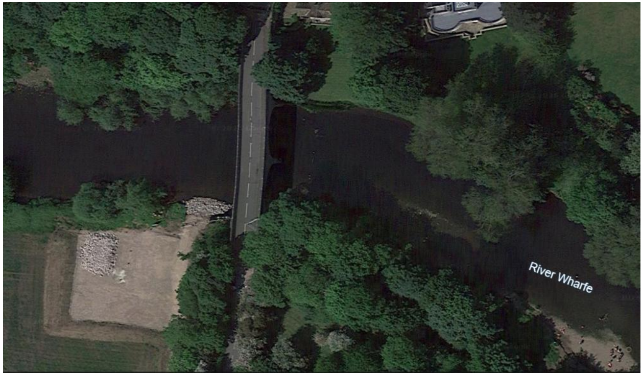
Figure 9 Construction platform for bridge repairs
