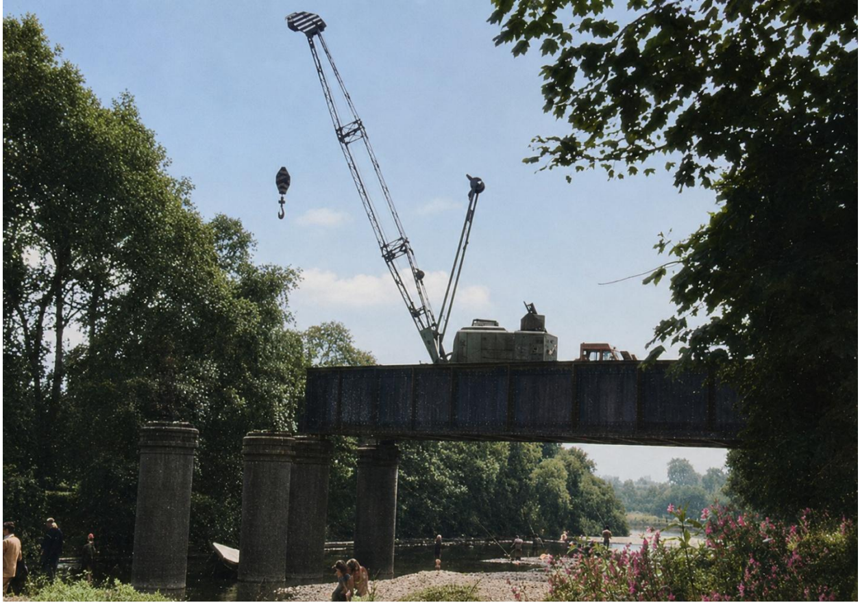
Figure 11 Dismantling the railway bridge
