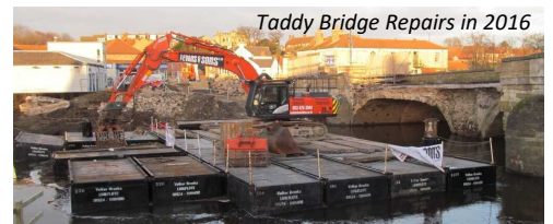
Taddy Bridge Repairs in 2016
